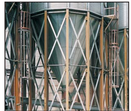
60 degree hopper slope
